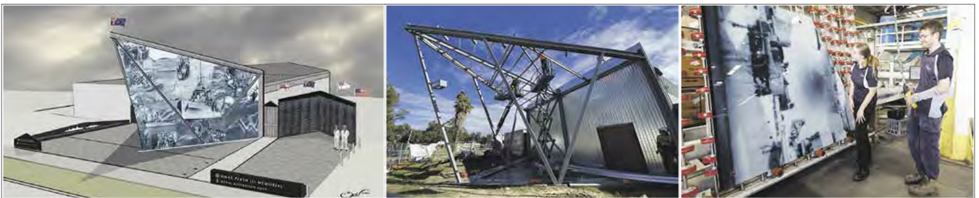
L-R; HMAS Perth I Memorial (Design concept) - The metal work for stage 2 nears completion - Joanne White, a graphic designer with Cooling Brothers and Matthew Rosveare casting an eye over a completed glass panel
