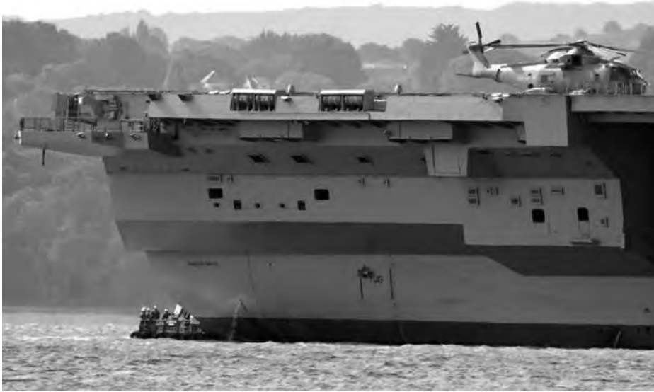
Divers Down Inspecting Damaged Prop Shaft of HMS PRINCE OF WALES (R09).
