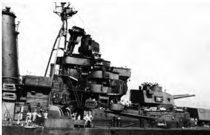
The damage to HMAS AUSTRALIA (II) bridge and foremast after air attack 21 October 1944 (image RAN).
