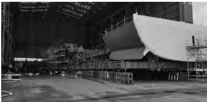
Hull of NUSHIP HMS GLASGOW being assembled - the first of the RN T26 GCF, April 2019.
