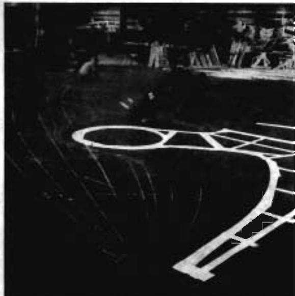
The mould staff of this British shipbuilding yard prepare mould butters and wooden templates from which plates and bulkheads are made, and rivet holes are marked.
