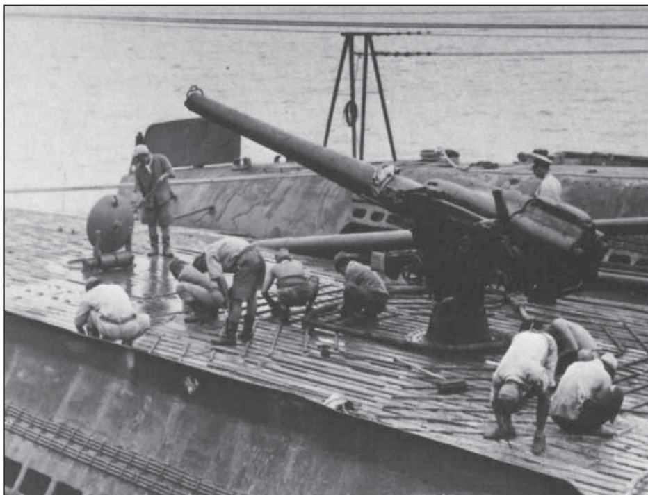
The standard Japanese submarine 5.5-inch (140mm) deck mounted gun. Even by today's standards this is a large gun.
