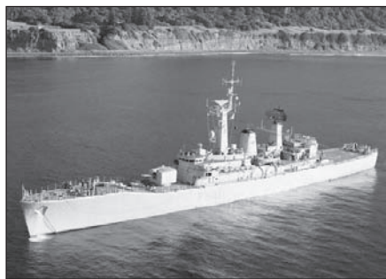
HMNZS CANTERBURY. Serious corrosion in hull and deck plating on the RNZN's aging frigate HMNZS CANTERBURY means the ship is no longer fully seaworthy. (RNZN)
