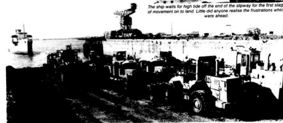
Well researched homework by Dawson Offshore had shown that once the front shoe on the cradle was in position, surprisingly little power would be required to edge the ship up its track. But when the ship became caught on the end of the slipway, it was sheer force which dragged her clear.
