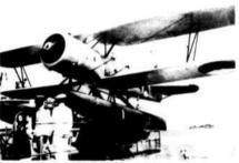
Fokker C VIIW aboard DE RUYTER, the only Dutch cruiser fitted with a catapult (Photo - RNN)
