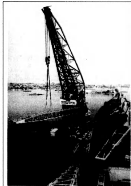
Heavy components of a 50 tonne crane to be employed in the construction of the Royal Australian Navy's new AOR are offloaded from the MV IRON CAPRICORN which carried it from Port Kembla as deck cargo. This ship building crane will supplement the present lifting capacity on Cockatoo Island. (Photo — Cockatoo Island).
