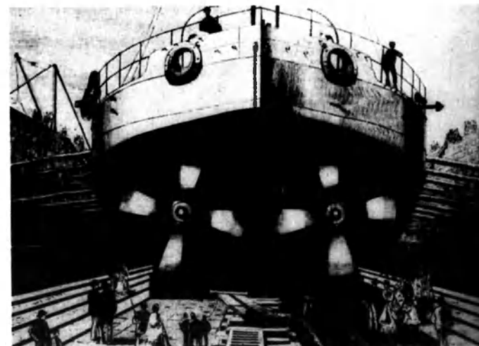
HMVS CERBERUS, dubbed the "Monster Class" by seamen, was the first iron-clad turret ship to be berthed in the Alfred Graving Dock. CERBERUS carried four ten-inch rifled muzzle-loading Armstrong guns and four one-inch Nordenfeldt quick-firers. Her engines had a nominal horsepower rating of 250 horses. CERBERUS was two-hundred-and-twenty-five feet long and forty-five feet wide. This picture is circa 1871.
