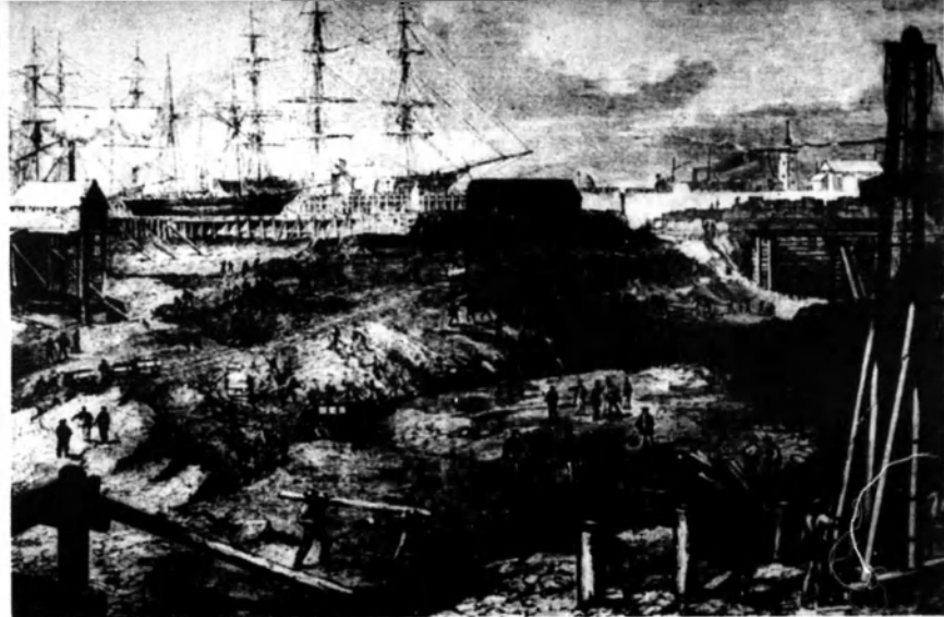
This drawing of Point Drake from 1865 shows men excavating the bed for the graving dock. First plans for the dock were made in 1853 by Captain Charles Ferguson, the Harbour Master. The coffer dam was finally constructed and pumped out in July, 1869.
