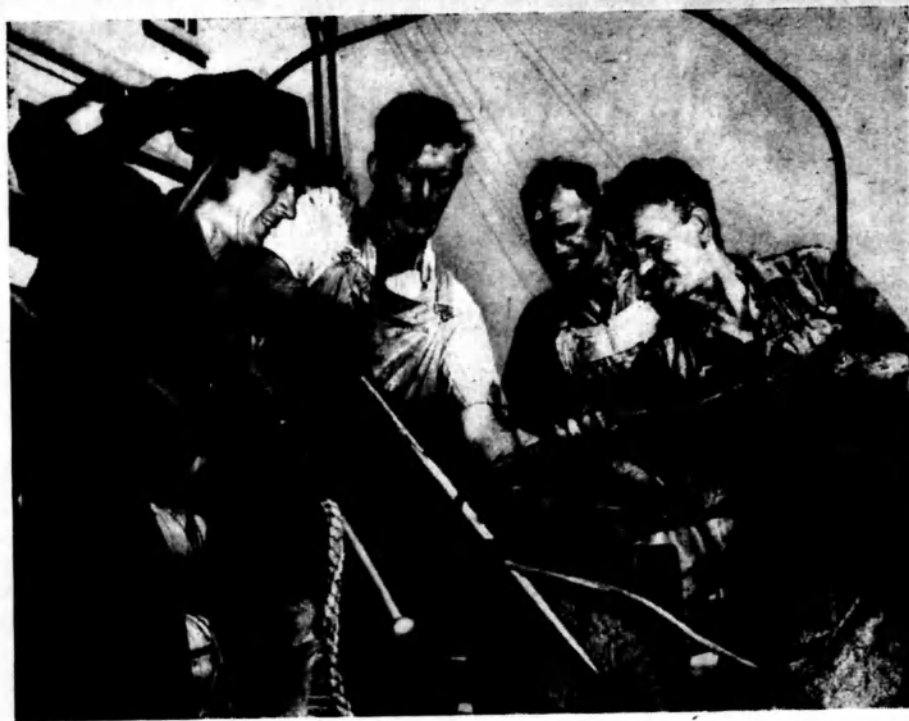
Riggers at Garden Island splicing the tow-rope which will be used to haul a Naval floating-dock from Newcastle to Williamstown, Victoria. The men are (left to right): Tom Formosa, Malcolm Macdonald, Bill Tarrant and Archie MacInnes. The tow-rope, 2,100 feet long, will be the biggest ever used on an Australian Navy job. The Naval tug, H.M.A.S. "Reserve," will tow the floating-dock to Sydney, where some small craft will be unloaded, then on to Williamstown.
