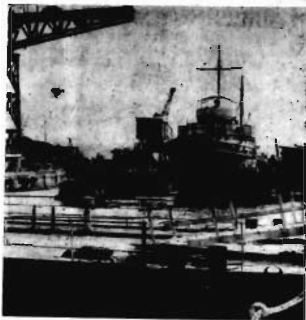
Here is a dock within a dock. To allow the naval tug Sprightly and a floating dock to be repaired simultaneously, the tug was placed inside the floating dock and the floating dock inside the Captain Cook graving dock.
