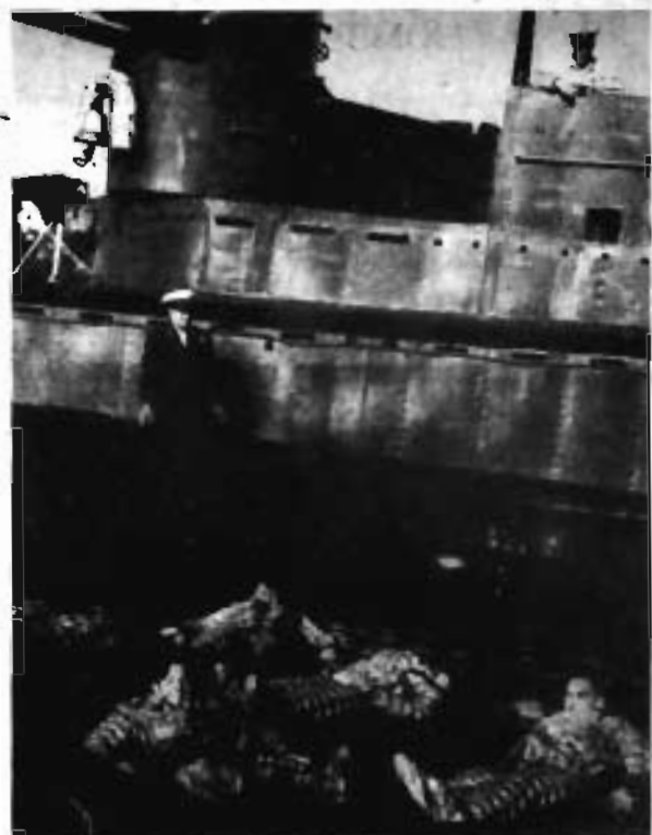
Crew of H.M.S. Telemachus testing inflated immersion suits. The suits are part of the submarine's rescue equipment and allow wearers to reach the surface more easily and keep afloat for long periods.
