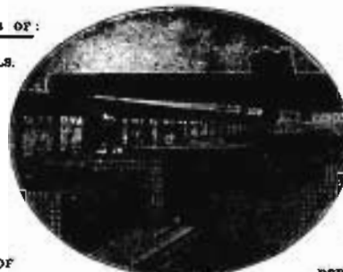
STACKING RAILS BY ELECTRIC MAGNET
