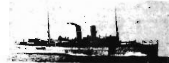
The R.I.M. "Northbrook," 5820 tons; 16 knots; six 4-inch; six 3-inch. "Dufferin" and "Hardinge" very similar.
